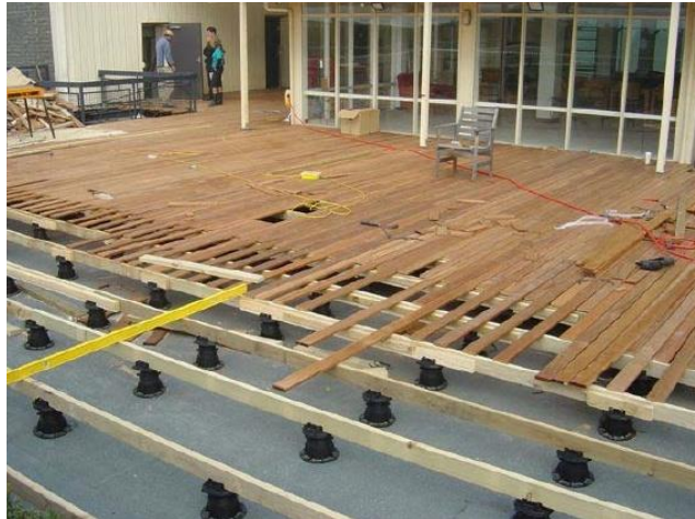
Figure 349 - The way of setting the Buzons
