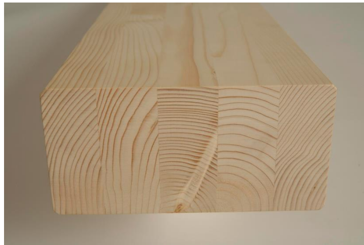
Figure 298 - Glued Laminated Timber Elements
