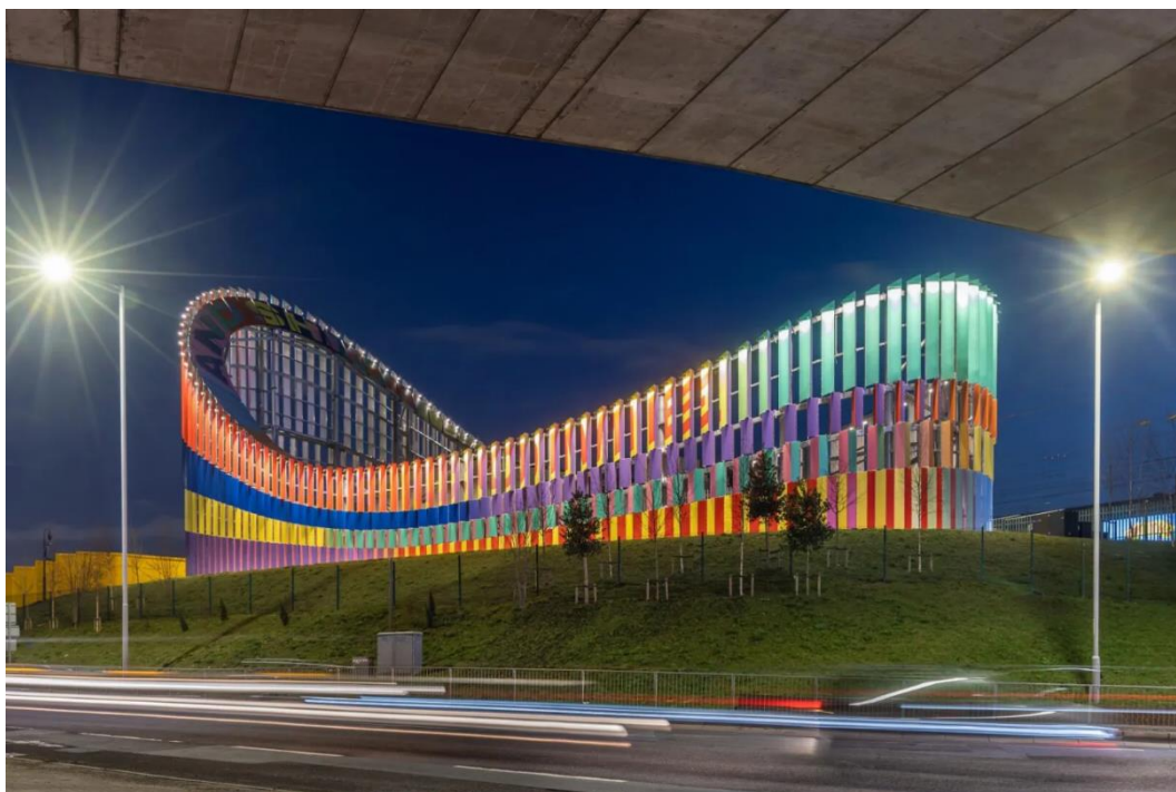
Slika 4.6 – Primarna transformatorska stanica Brent Cross Town, London [25]
